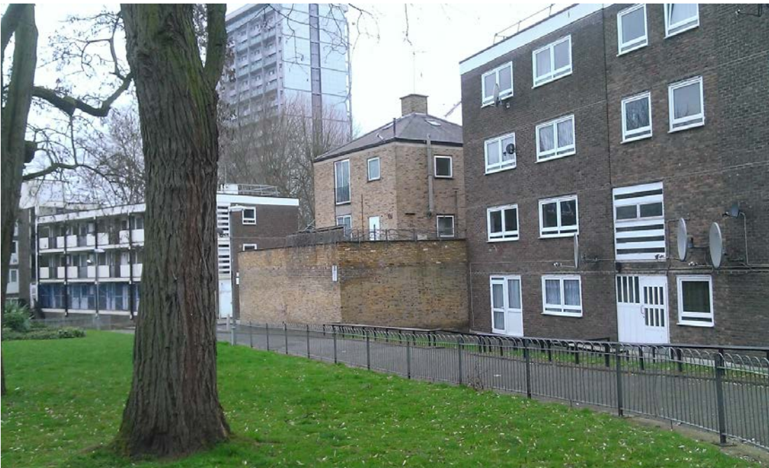
View of front of site from Lord Hills Road (top) and rear elevation (bottom).
